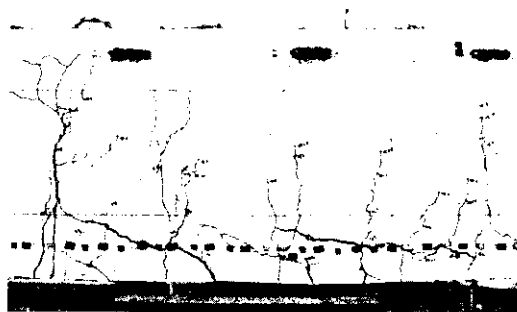
Photo. 3 Fracture of lapped splice on Ft1
