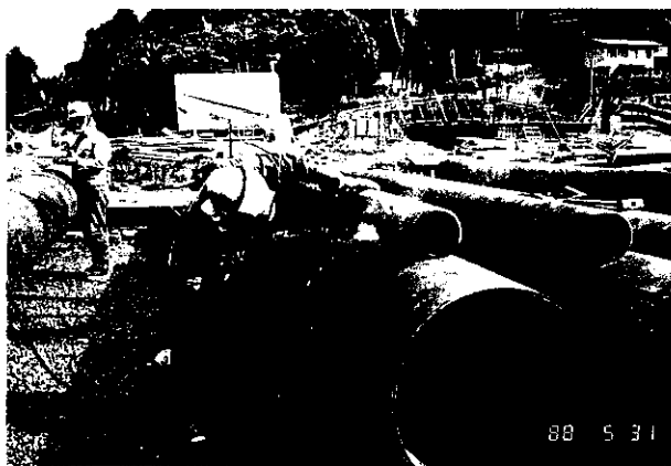
Photo 1 Site fabrication of interlocked steel pipe piles
